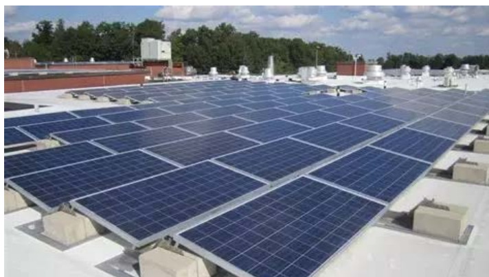
Multicrystalline plant on fixed structures
