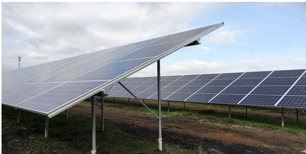
Multicrystalline plant on fixed structures
