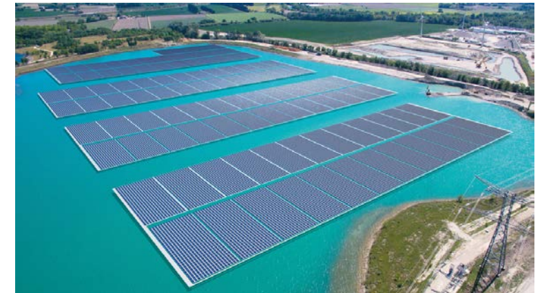
Europe's largest floating solar system, located in Piolenc (France), powered by 17MW of Trina Solar PV modules. | Photo: Akuo Energy
