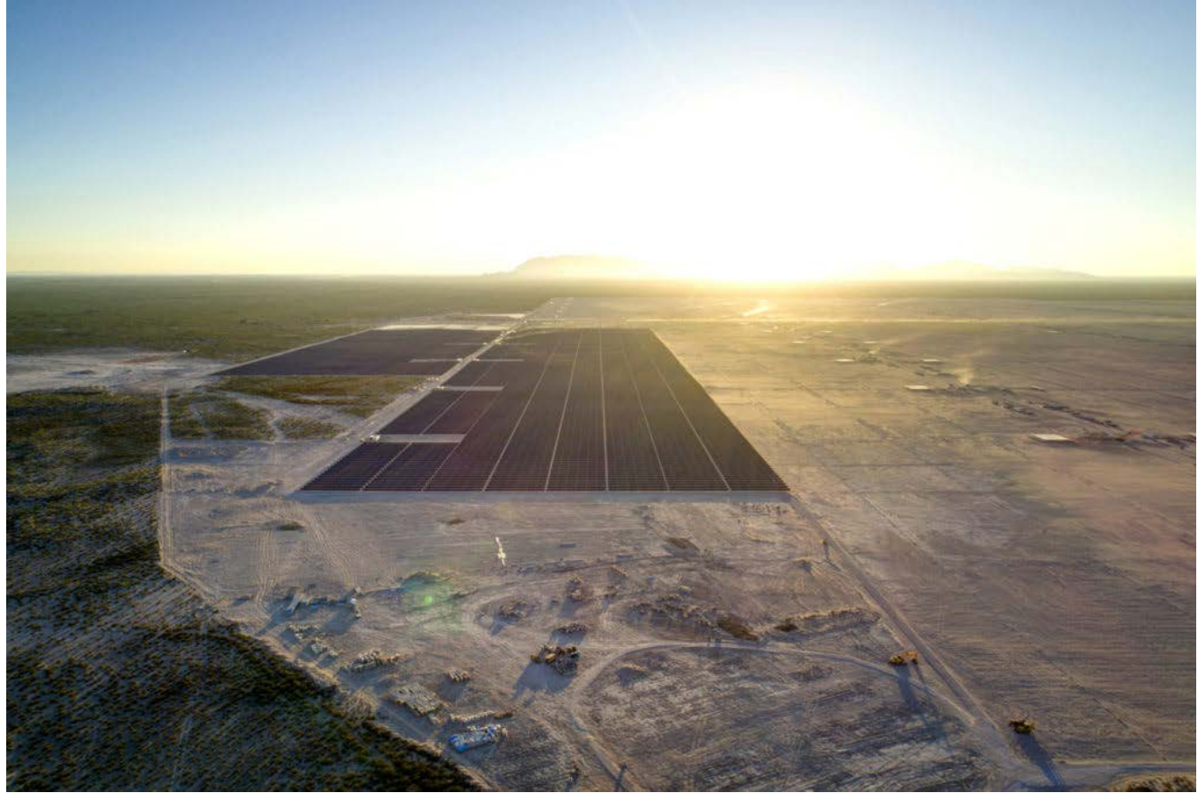
With 2,300,000 PV modules, Enel's Villanueva project is currently the largest solar plant in the Americas. Image: Secretaría de Energía/Gobierno de México
